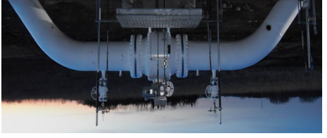
DAPL exposed at shut-off valve
