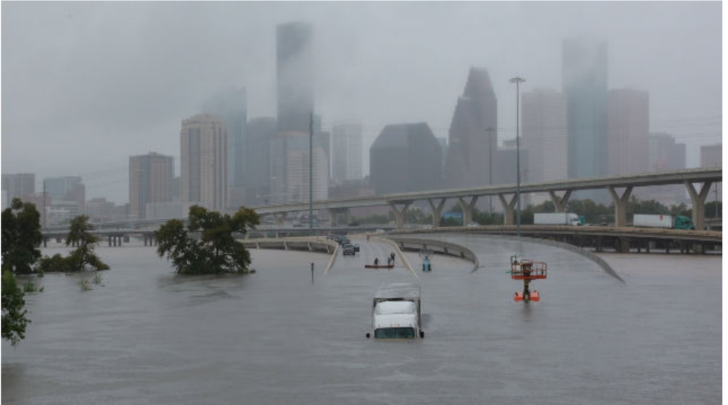
Hurricane Harvey — Houston, TX, US — August 2017
