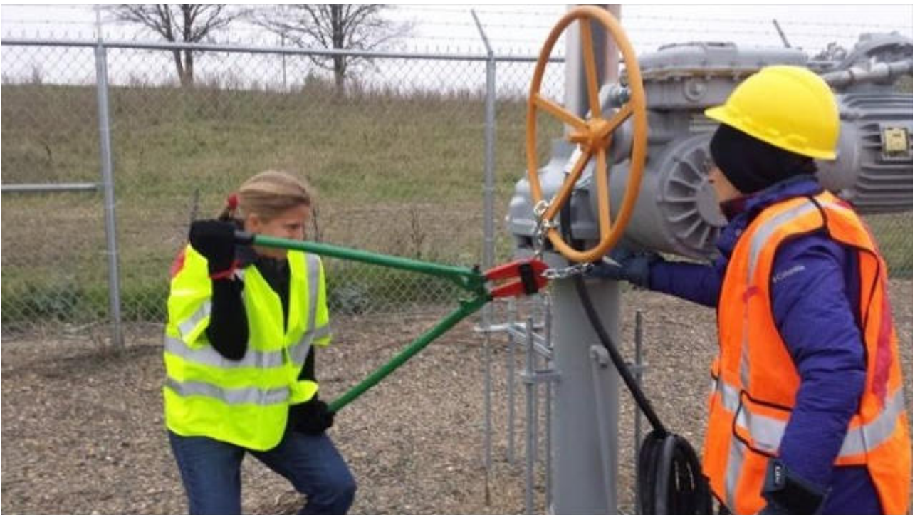
Valve Turners shutting down a pipeline
