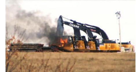
Sabotage of DAPL pipeline construction
